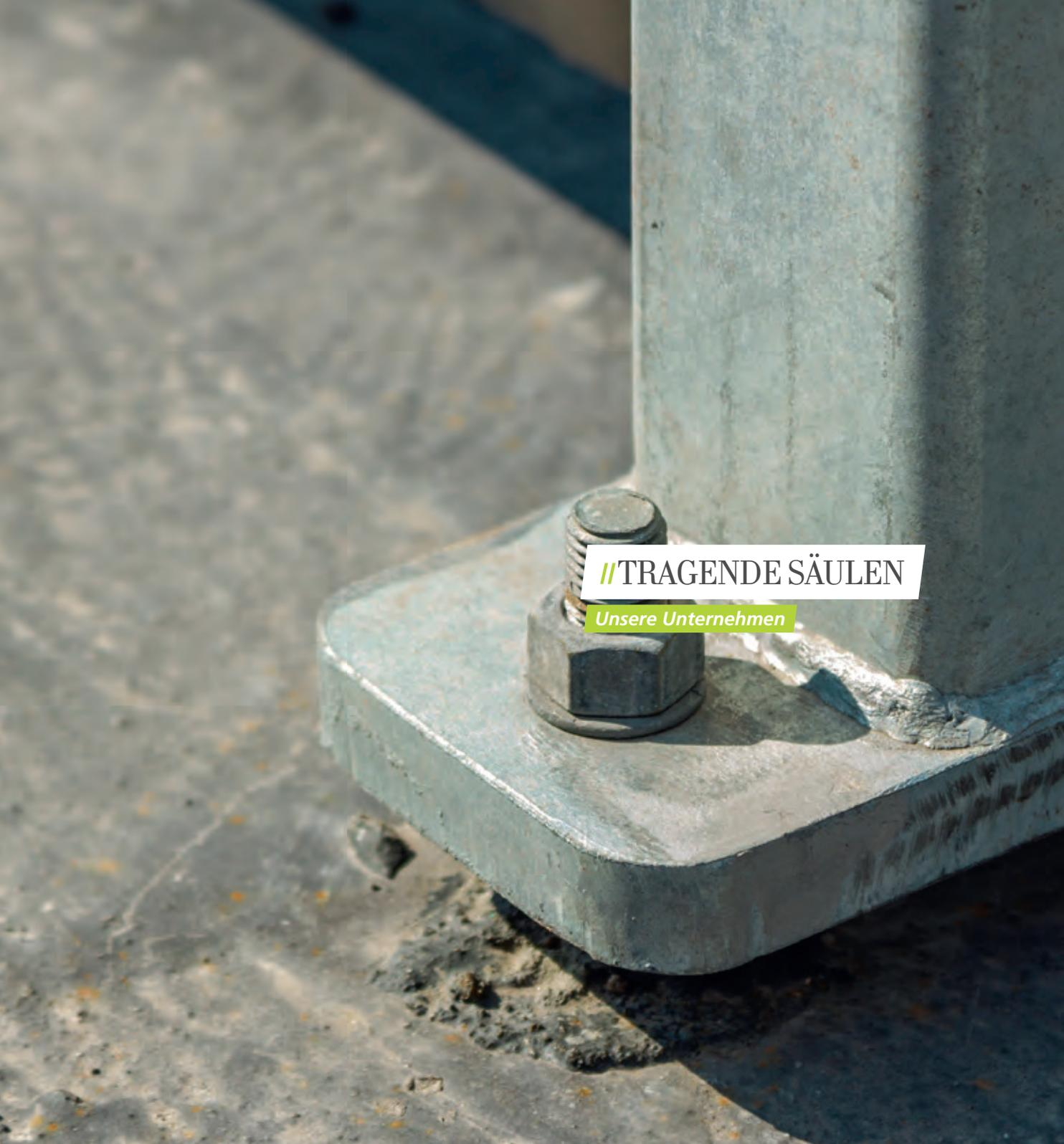
A close-up photograph of a heavy-duty metal bolt and nut securing a steel column base to a concrete floor. The bolt is positioned vertically, passing through a hexagonal nut and a thick metal plate. The steel has a weathered, greyish-blue patina. The background is a blurred concrete surface.
